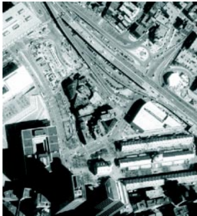
Figure 3. Downtown Boston, 1995: as construction begins on the depressed Central Artery Tunnel.
